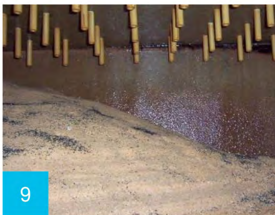
Figure 7 Algae growth – risk of cyanotoxin production; uneven filter backwash
